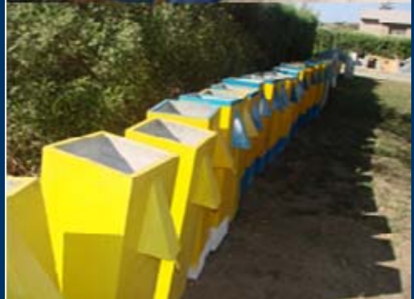
Biosand water filters being installed to meet the clean drinking water need in Chipulukusu
