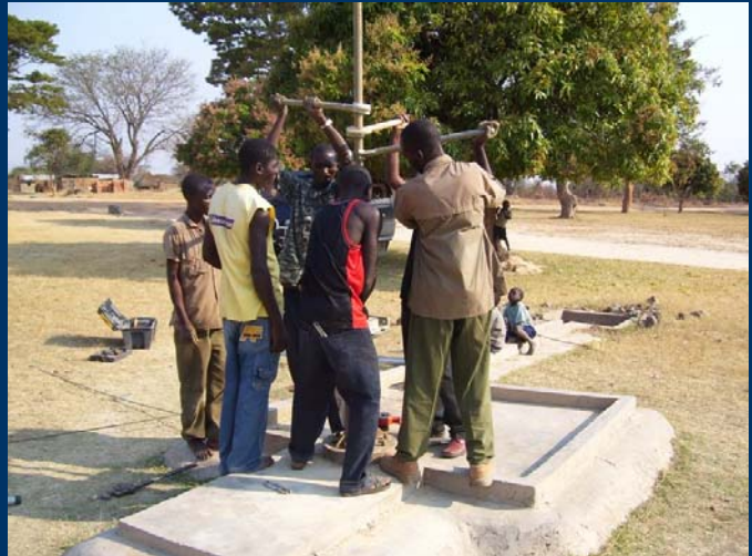
Team repairing the well at Katuba Basic School.
